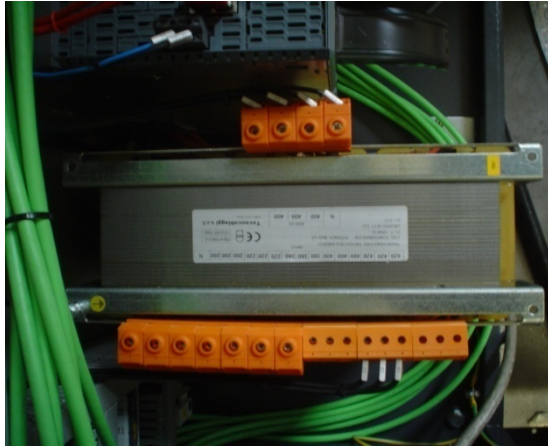
Figure9:Connecting to the power 电源连接
