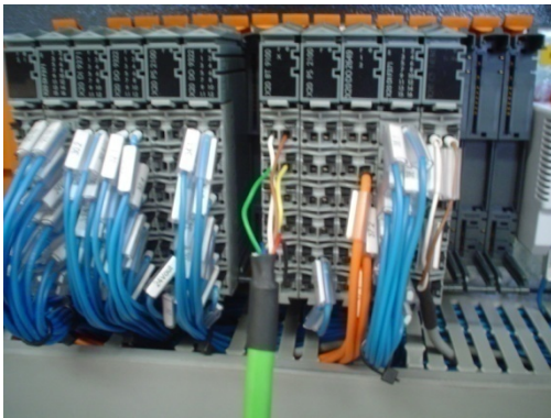
Figure 41: Connection of the system management encoder 系统管理编码器的连接
