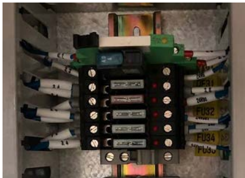
Figure79:Replacing fuses 更换熔断器
