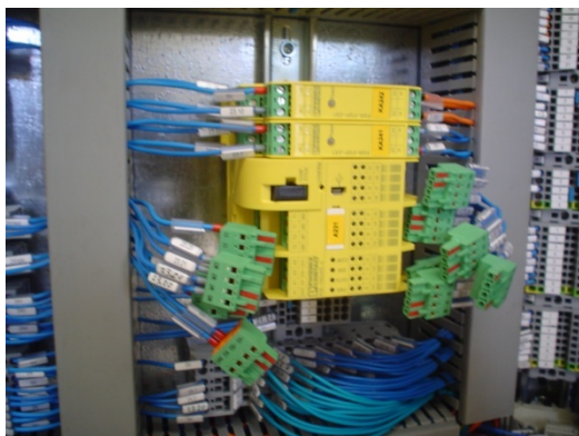
Figure 27: Replacing the safety PLC 更换安全 PLC
