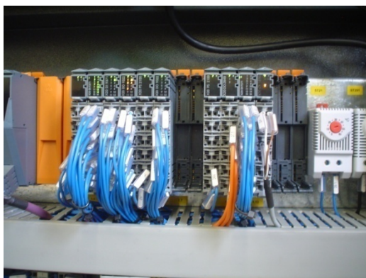
Figure37: Connection of the system management encoder 系统管理编码器的连接
