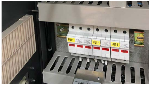
Figure78:Replacing fuses 更换熔断器
