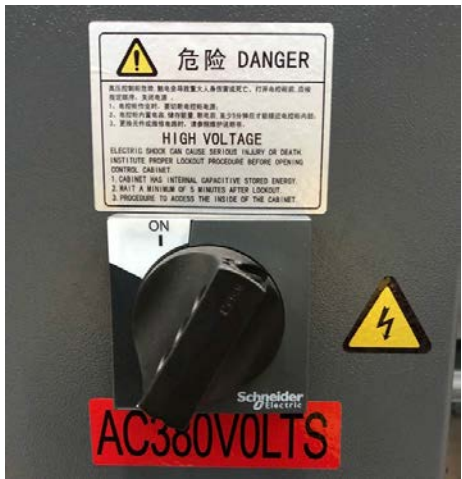
Figure63:Electrical Cabinet ON/OFF switch 电柜 ON/OFF 开关
